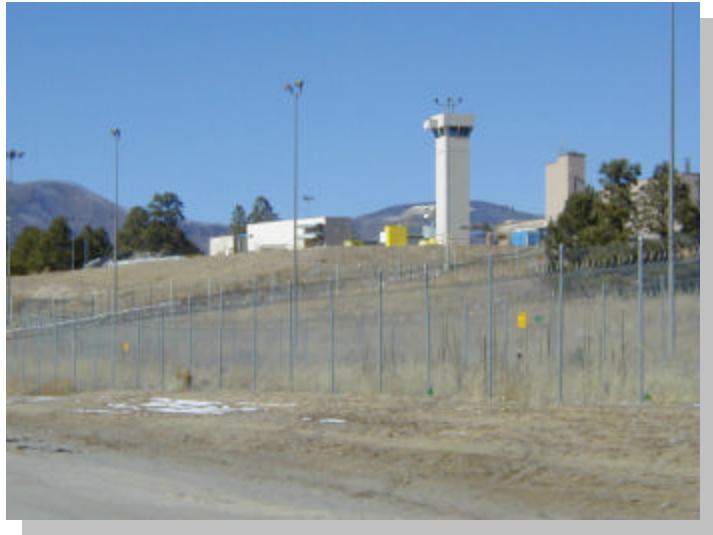
LOS ALAMOS NATIONAL LABORATORY'S PLUTONIUM FACILITY
